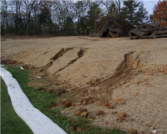
Active erosion is controlled with silt sock
