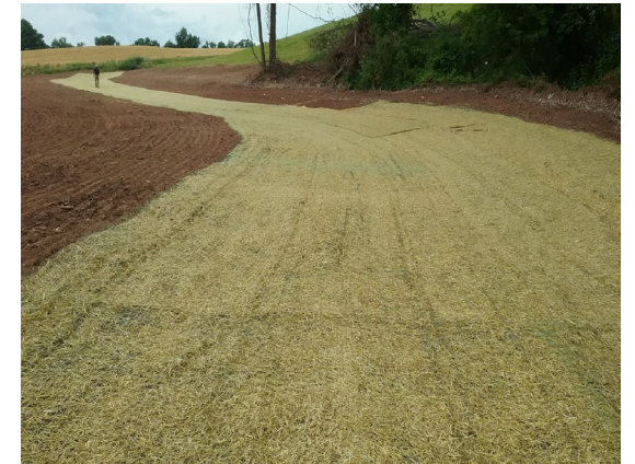
Newly constructed grass waterway
