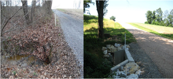
Culvert crossing replaced on Bittle Road, Germany Twp from a 30 inch pipe to 9 foot wide box culvert
