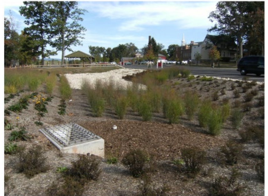
Extensive landscaped rain garden - before
