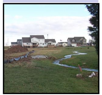
LEAVE IT GREEN! Practice erosion control by keeping the soil covered with vegetation, which will not allow the soil to erode easily. Minimize amount of disturbance at any given time. Plan your grading around the growing season for establishing vegetative cover.
