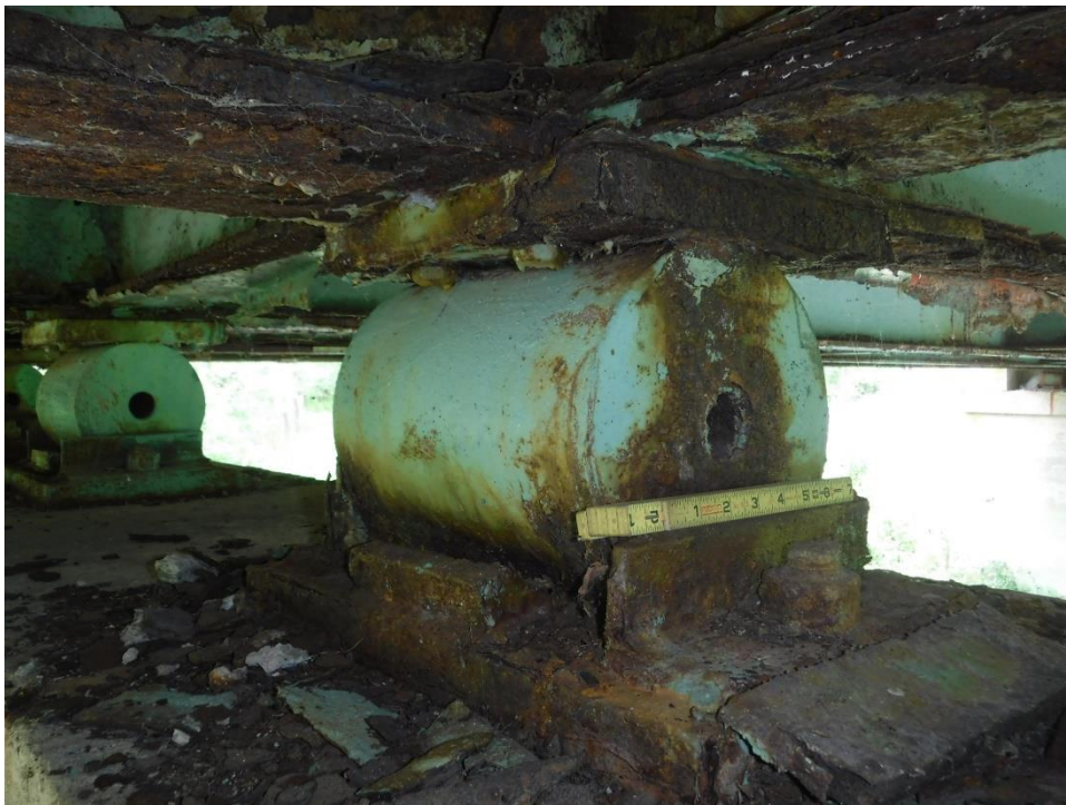
Photo No. 12 - Typical condition of expansion bearing at pier. Beam 4 bearing shown.
