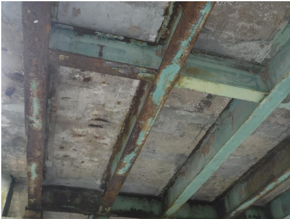
Photo No. 8 – Spalls with exposed reinforcement bars along left overhang, Span 1.
