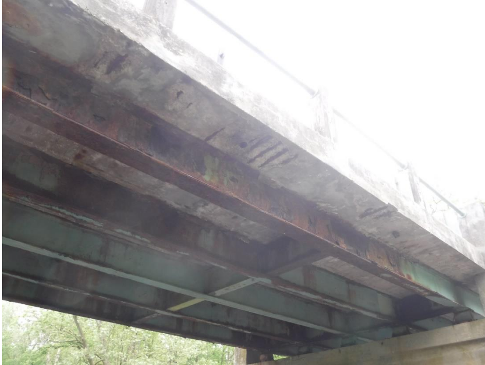
Photo No. 7 – Right overhang, Span 1. Note spalls with exposed reinforcement.
