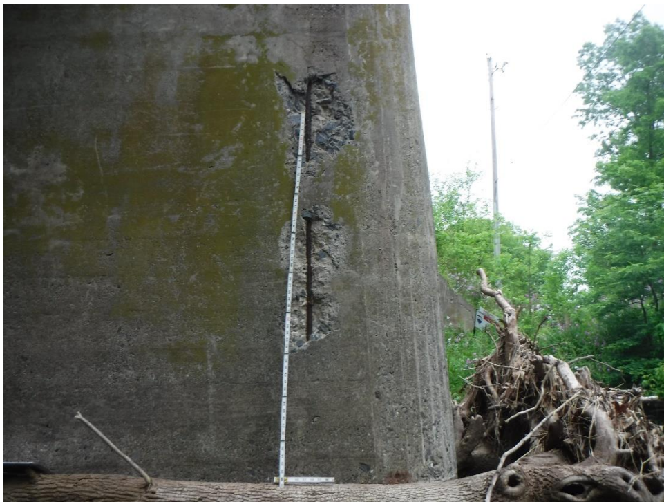
Photo No. 14 – Spall with exposed bar on pier at far right.
