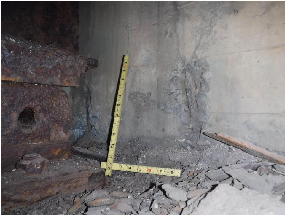
Photo No. 13 –Two spalls with exposed reinforcement bars on far abutment backwall.
