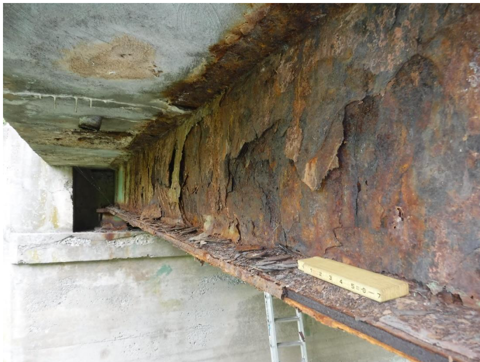
Photo No. 10 – Severe corrosion to outside face of right fascia beam, Span 1.
