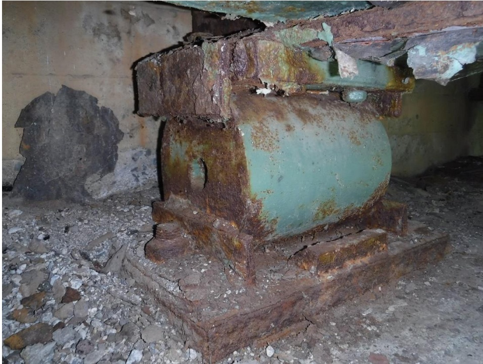
Photo No. 11 – Typical condition of expansion bearing at far abutment.
