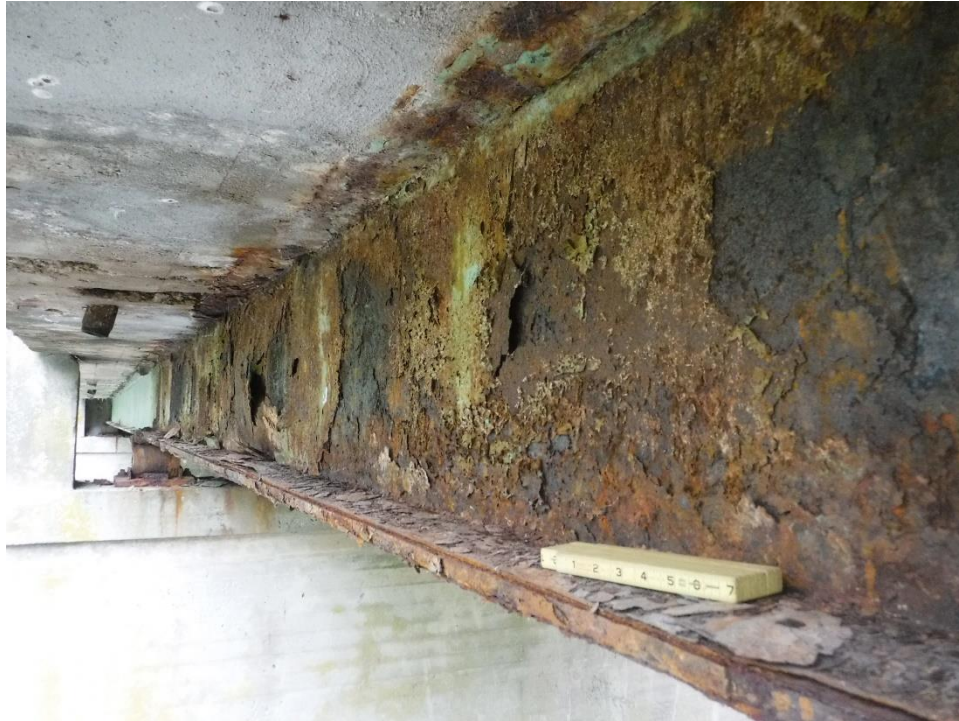
Photo No. 9 – Severe corrosion to outside face of left fascia beam, Span 1.
